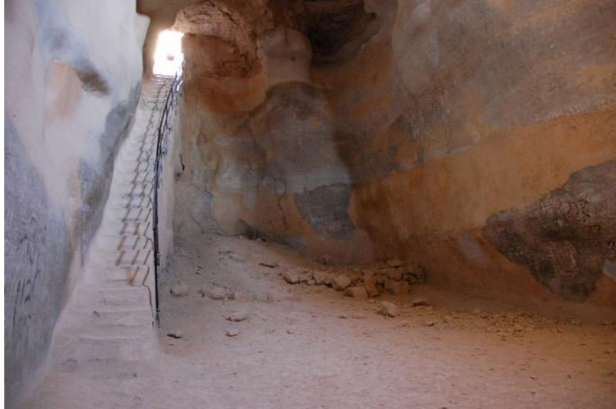
Figure 2: Large water cistern at Masada. This figure shows one large water cistern that illustrates its enormous size.
