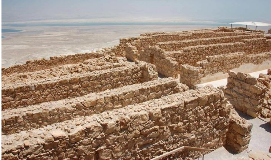
Figure 2: The Store-houses at Masada. According to Josephus, these store-rooms were used to store large quantities of grain, fruit, oil, and wine, all of which had remained fresh even though stored there for a hundred years. Weapons were also stored there in great quantities.
